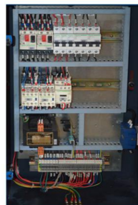
CE electric box
