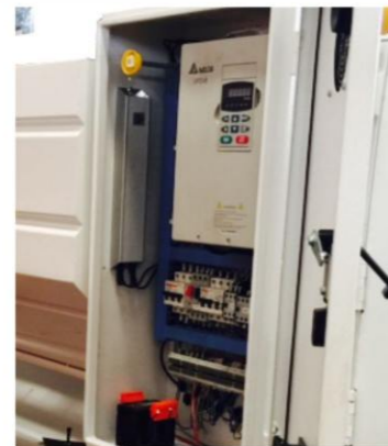
Inverter and variable frequency motor
